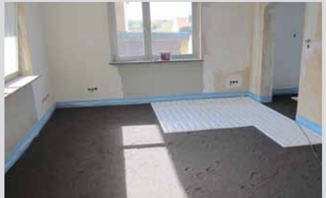
Laying of system element
