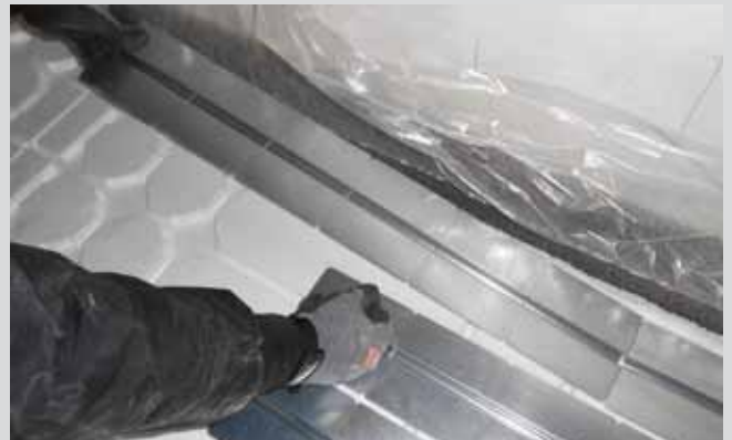
Installation of heat conducting steel sheets
