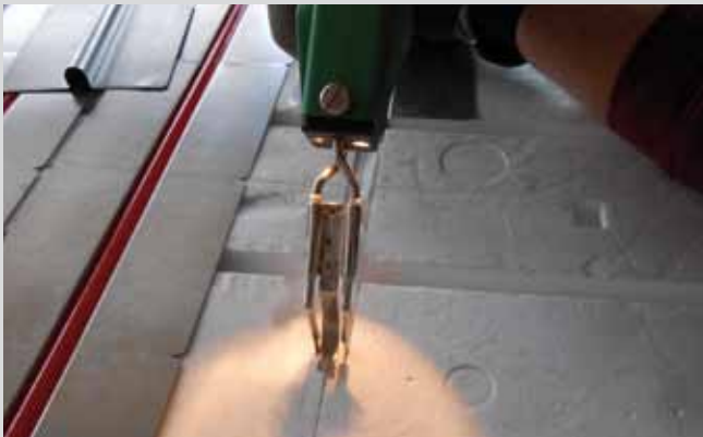
Required extra pipe channels such as connecting pipes are made by filament cutter.
